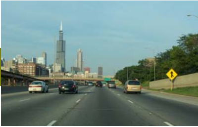
Eisenhower Expressway resurfacing
