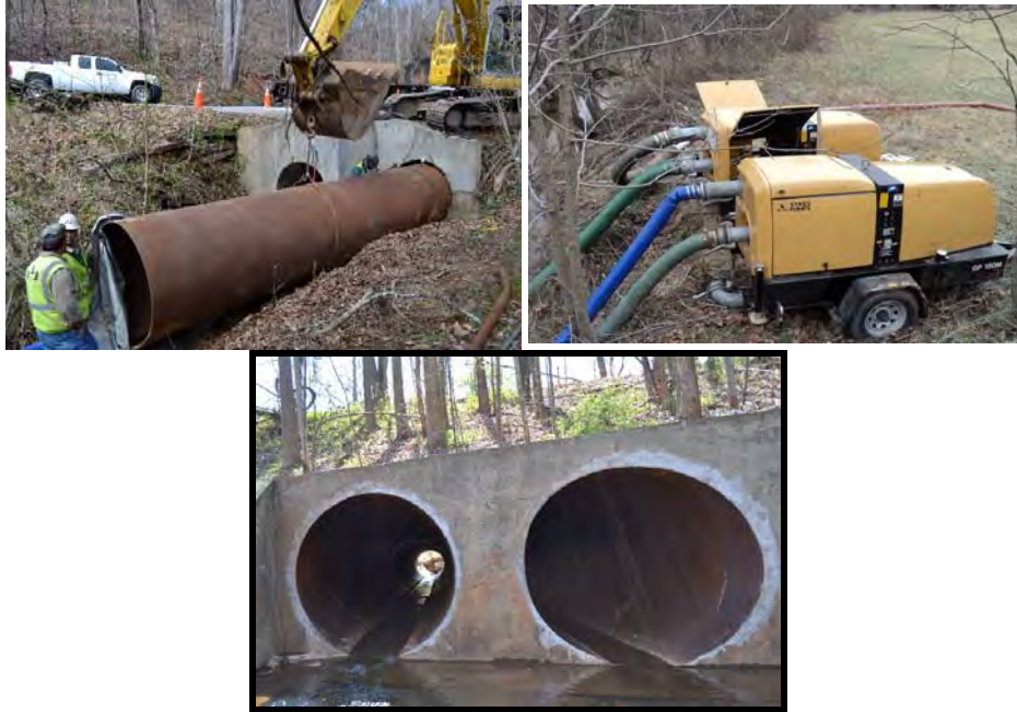
Figure 2 Sequence of installation
